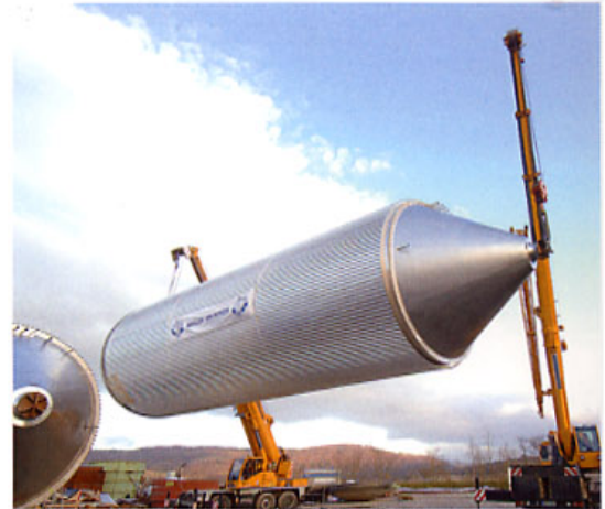
Installation of a zyl.-kon fermentation and storage tank
